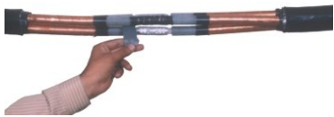
Application of Stress Grading pad
