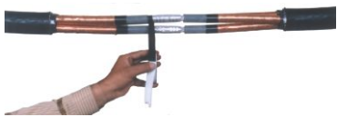
Application of semiconducting tape
