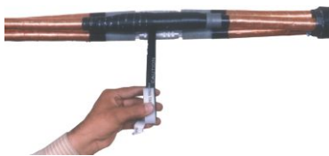
Application of Self Amalgamating Insulating Tape
