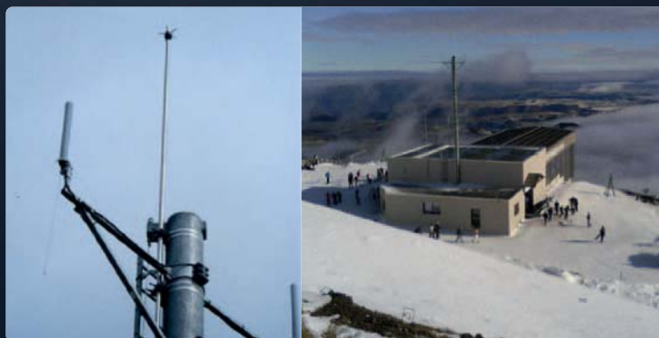
ESE air terminal in extreme climatic conditions
